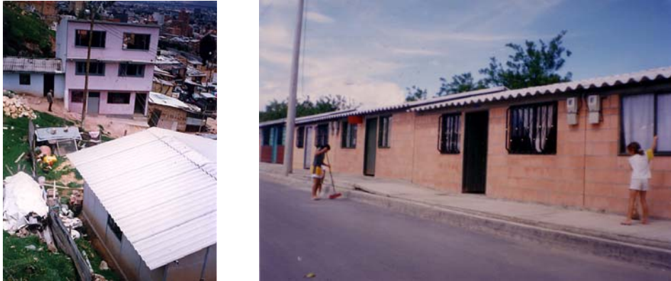
Fig. 2. Left: Informal settlement in Bogotá showing 4 different stages in the housing evolution process: from a shack made of scrap wood to a three storey unit made of concrete and masonry. Right: 1-storey units in El Cantarito. Despite that higher densities were obtained and infrastructure was provided, few months after the project was finished, users had already modified the rigorously standardized facades to personalize them with colours and finishes.
