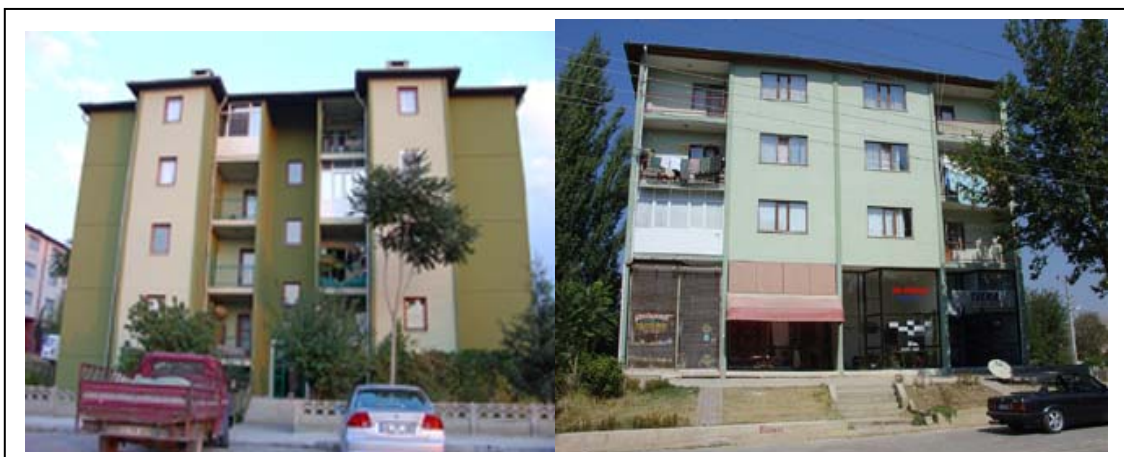
Two types of post-disaster houses in center of Dinar
