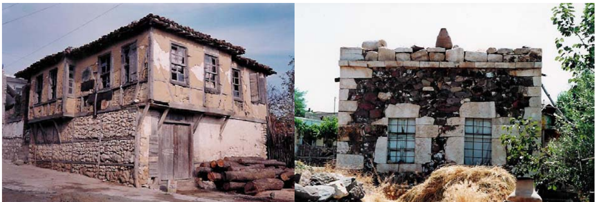
Figure 5. The timber frame construction with masonry infill and masonry construction examples of traditional houses.
