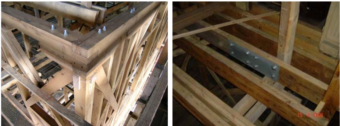
Figure 12. Reinforcing the joints of the timber buildings using mechanical fasteners (Can Binan's archives)
