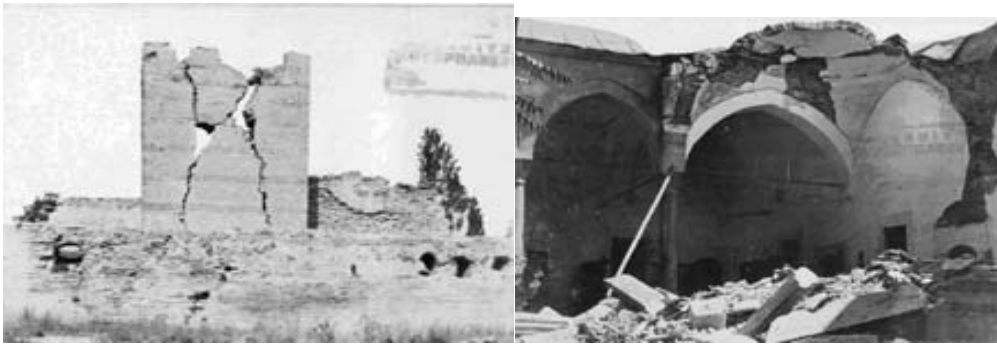
Figure 1. 1894 earthquake in Istanbul
