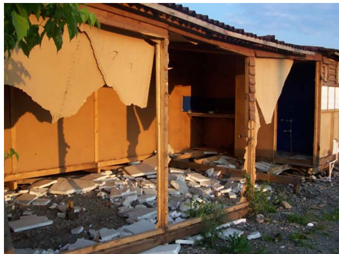
Figure 4 View of the temporary houses after evacuation
