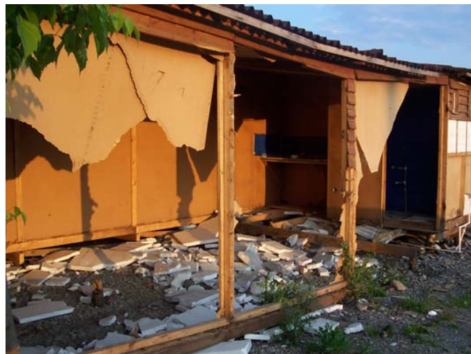
Figure 4 View of the temporary houses after evacuation
