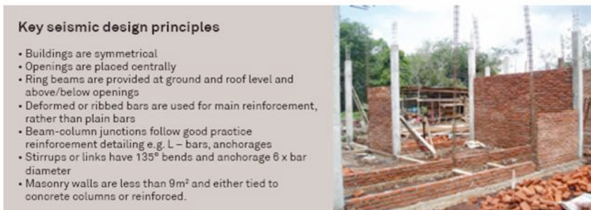
Fig. 5. Brick Infill Walls Engineering Advice
