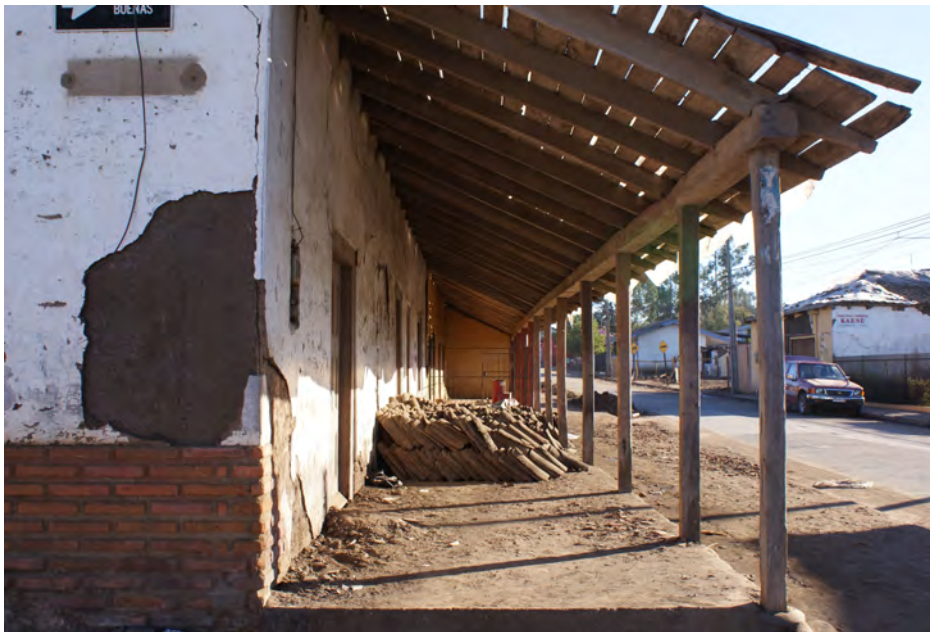
Figure 1. An adobe house affected by the 2010 earthquake in the heritage area of Chanco. Source: B. Devilat, April 2010.
