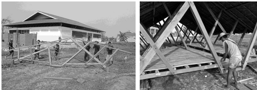
Figure 5: Left and Right: Temporary Dormitories assembly process. Source: http://openarchitecturenetwork.org/ .
