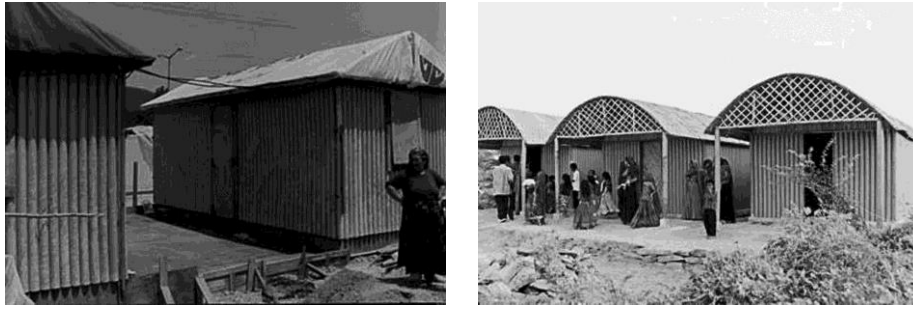
Figure 4: Paper Log Houses. Left: Transformation of two units into a three-room dwelling using the space between concrete. Source: Johnson, 2008; Right: Solution used in Gujarat, India. Source: http://www.shigerubanarchitects.com/ .
