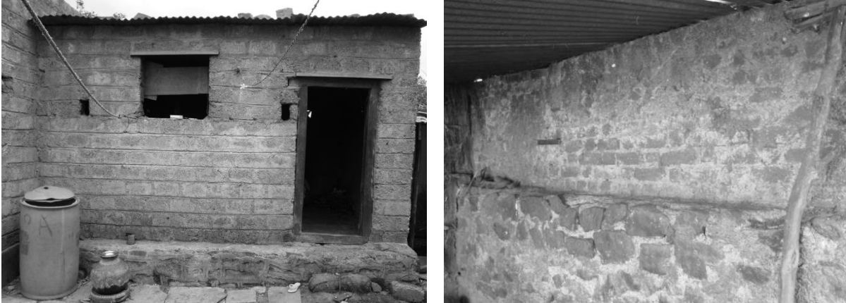
Figure 15: Left: Muslim farmers' house in Gubbal made of independent brick structure of high walls without horizontal tie band; Right: Dhangar house in Gubbal made of hybrid material walls. Source: Authors, 2011.
