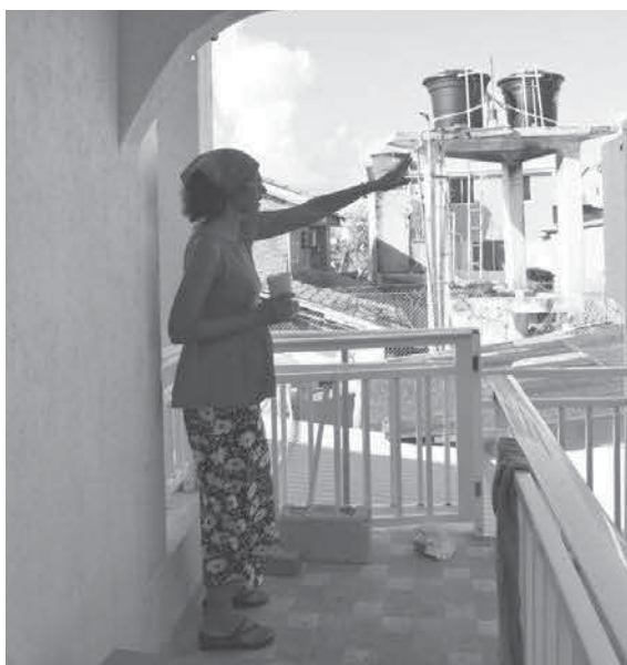
Figure 9: Carson's Place 2's domestic rainwater harvesting system. Source: The Authors
