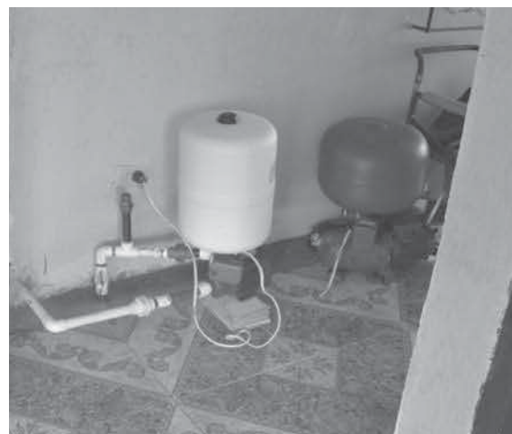
◀ Figure 6: Justina's Place's domestic rainwater harvesting system. Source: The Authors
