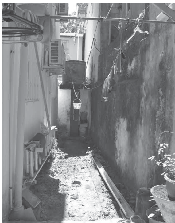
Figure 5: Cli's Place's domestic rainwater harvesting system. Source: The Authors
