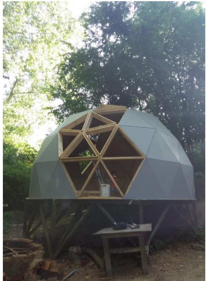
Fig. 9. Plywood plates painted with waterproof paint. Source: Entorno Educador school.
