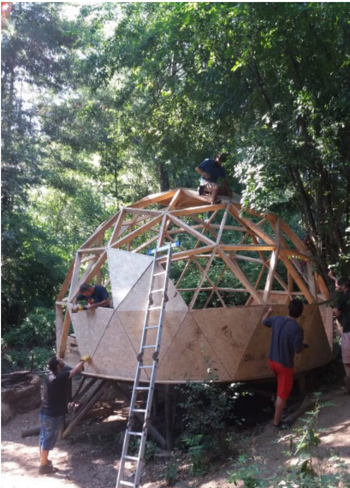
Fig. 8. Installation of the structural plywood plates. Source: Entorno Educador school.
