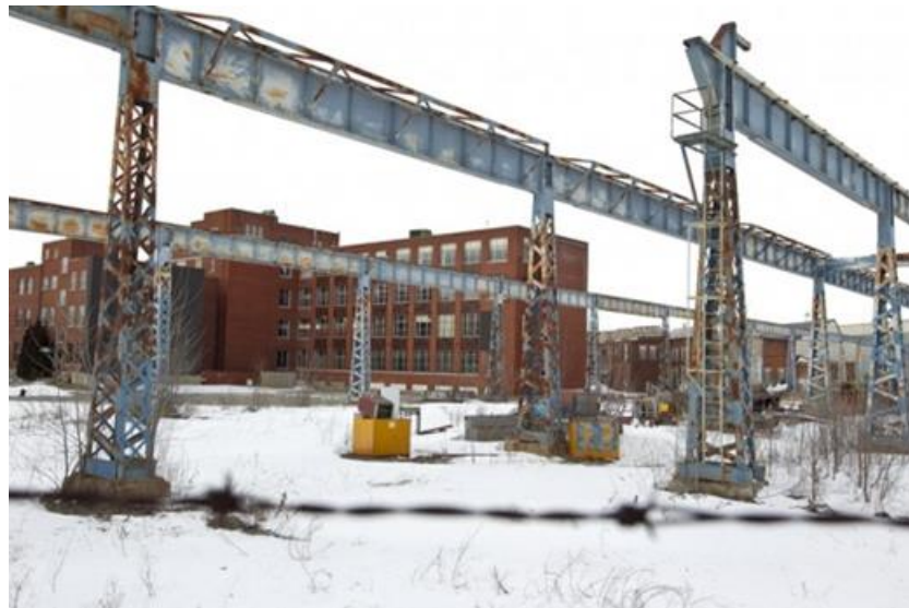
Figure 5: Dominion Bridge Company (Photo: Alain Roberge)
